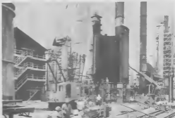
Lago's newest heavy equipment asset is this American crane, with 60-ton capacity and a 100-ft. boom. Here it sets part of the new furnace for No. 9 Pipestill in place.
